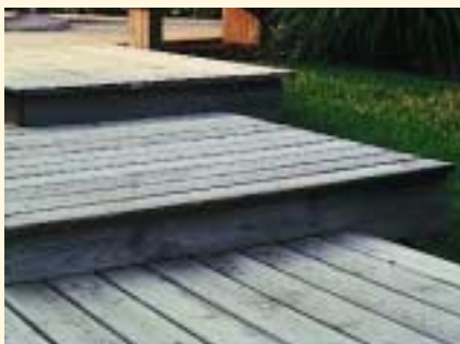
Pressure-treated wood was, until recently, the material of choice for constructing decks, stairways, raised beds, and other garden structures.
